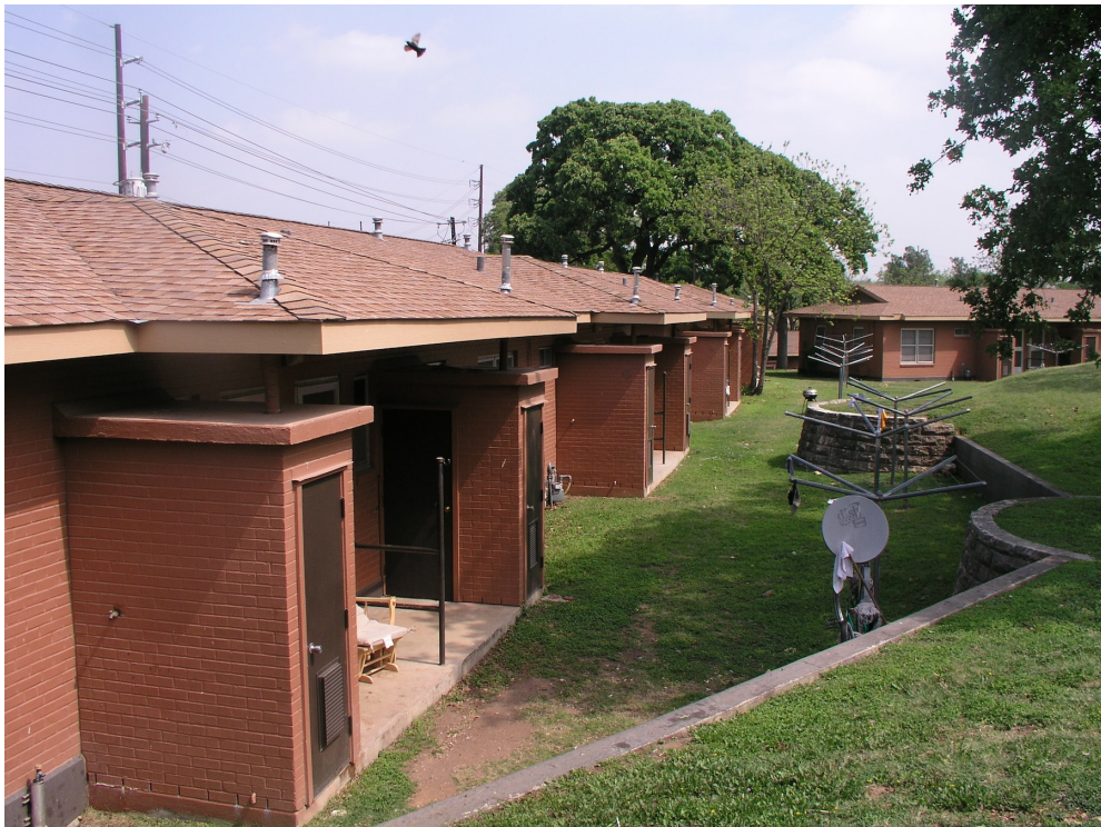
Photo 20: Water Heater Closets, Clotheslines, Terracing, and Retaining Walls, April 16, 2013
